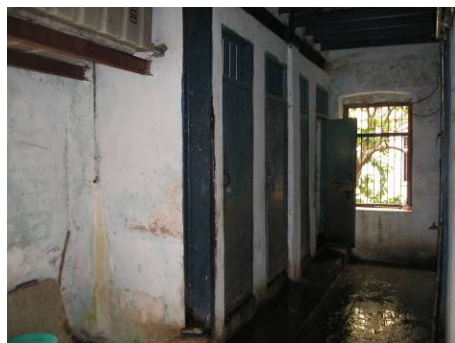
Fig.22: Common toilets, case study 1 chawl at Naigaon.
