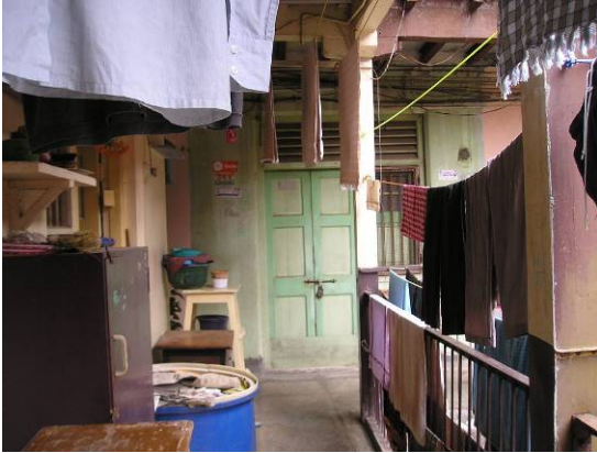
Fig.48: Multifunctional corridor, case study 1 chawl at Naigaon.
