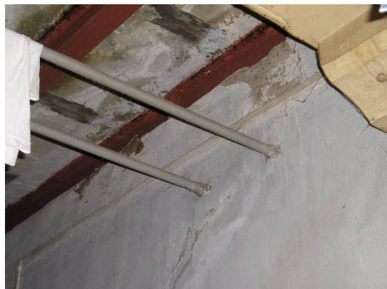
Fig.32: Steel joists, case study 1 chawl at Naigaon.
