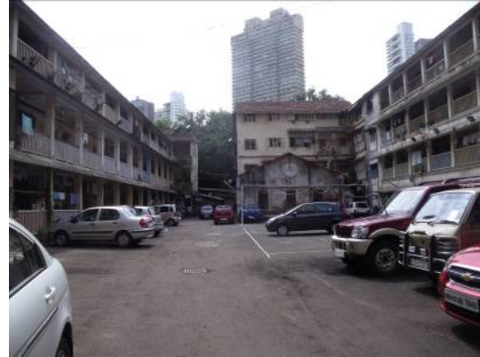
Fig.21: View of chawl buildings and courtyard as seen from the entrance to case study 2 chawl at Grant Road.
