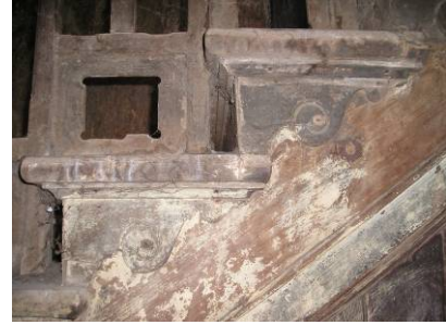
Fig.35: Rusted railing of the staircase, chawl at Naigaon. Source of Image: Taken by Author
