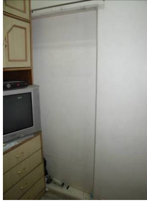
Fig.50: Niche in the living room wall created when the door leading to the neighbor's house was taken out, case study 2 chawl at Grant Road.
