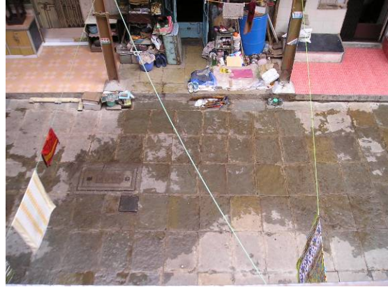
Fig.49: View of courtyard from second floor corridor, case study 1 chawl at Naigaon.
