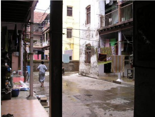
Fig.29: View of courtyard seen from the entrance, chawl at Naigaon.
