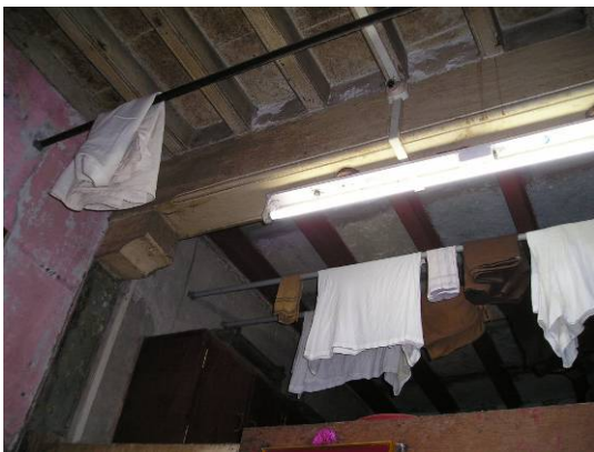
Fig.31: Timber and steel joists, case study 1 chawl at Naigaon.
